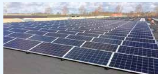
Installation of solar panels at Gits
