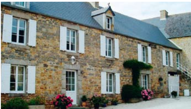
France - Zendow windows with Kiuzo shutters
